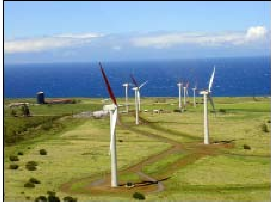
Hawi Renewable Development LLC Wind Farm at Upolu Point near Hawi on the Island of Hawaii. Source: Hawaiian Electric Light Company via NREL Photo Information Exchange.
